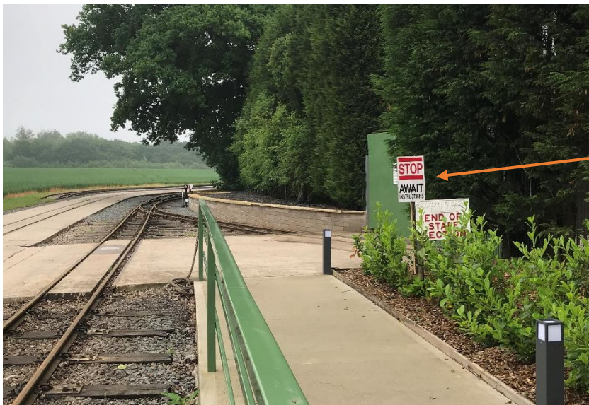
These pictures show the new point indicators and new stop board
